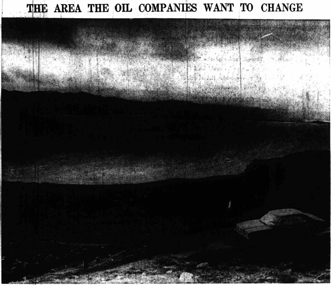
STORM clouds over Loch Carron and Loch Kishorn, south-west Ross-shire. Immediate left foreground is the proposed site for the Howard/Doris partnership, who want to build a series of concrete production platforms for North Sea oil and gas.
