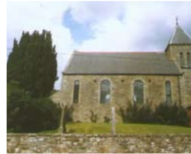
The stone built church at Falstone in Northumberland
