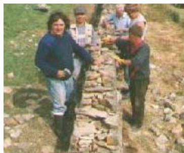
Constructing a stone wall. Note the rubble in the middle
