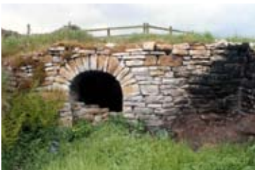
A stone built tunnel which once supplied air to a lead mine
