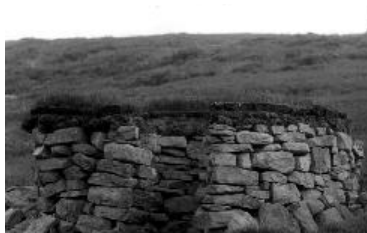
Note how the butt is built with stone and the turf laid on top helps to protect the wall
