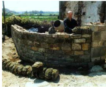
A stone wall being built at Slaley
