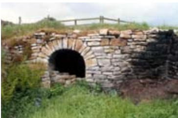
A stone built tunnel which once supplied air to a lead mine
