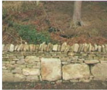
A stone wall in the north with large stones placed in the wall
