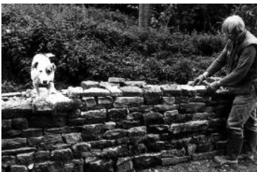
A stone wall being built near Haydon Bridge in Northumberland
