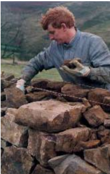
The heart of the wall being filled with small packing stones.
