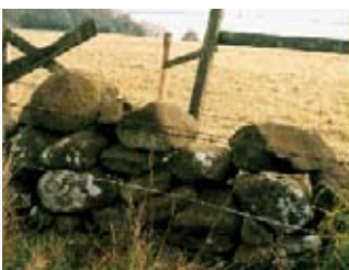
Part of a stonewall in Galloway constructed with round rough stones - probably collected from fields or riverbeds.
