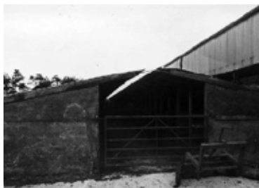
Cow kennels. Note how low the building is with an opening at the top for ventilation
