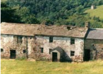
Some old farm buildings. Note the big stone slates on the roof
