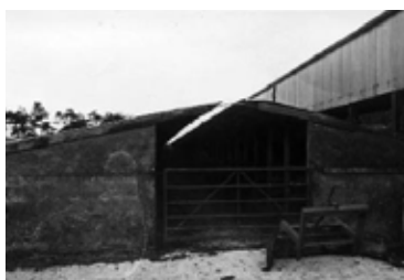
Cow kennels. Note how low the building is with an opening at the top for ventilation
