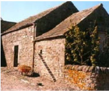
An old stone farm building. Note the steps where hens would walk up into the loft.
