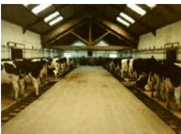
A double sided cow byre with automatic muck scrapers.
